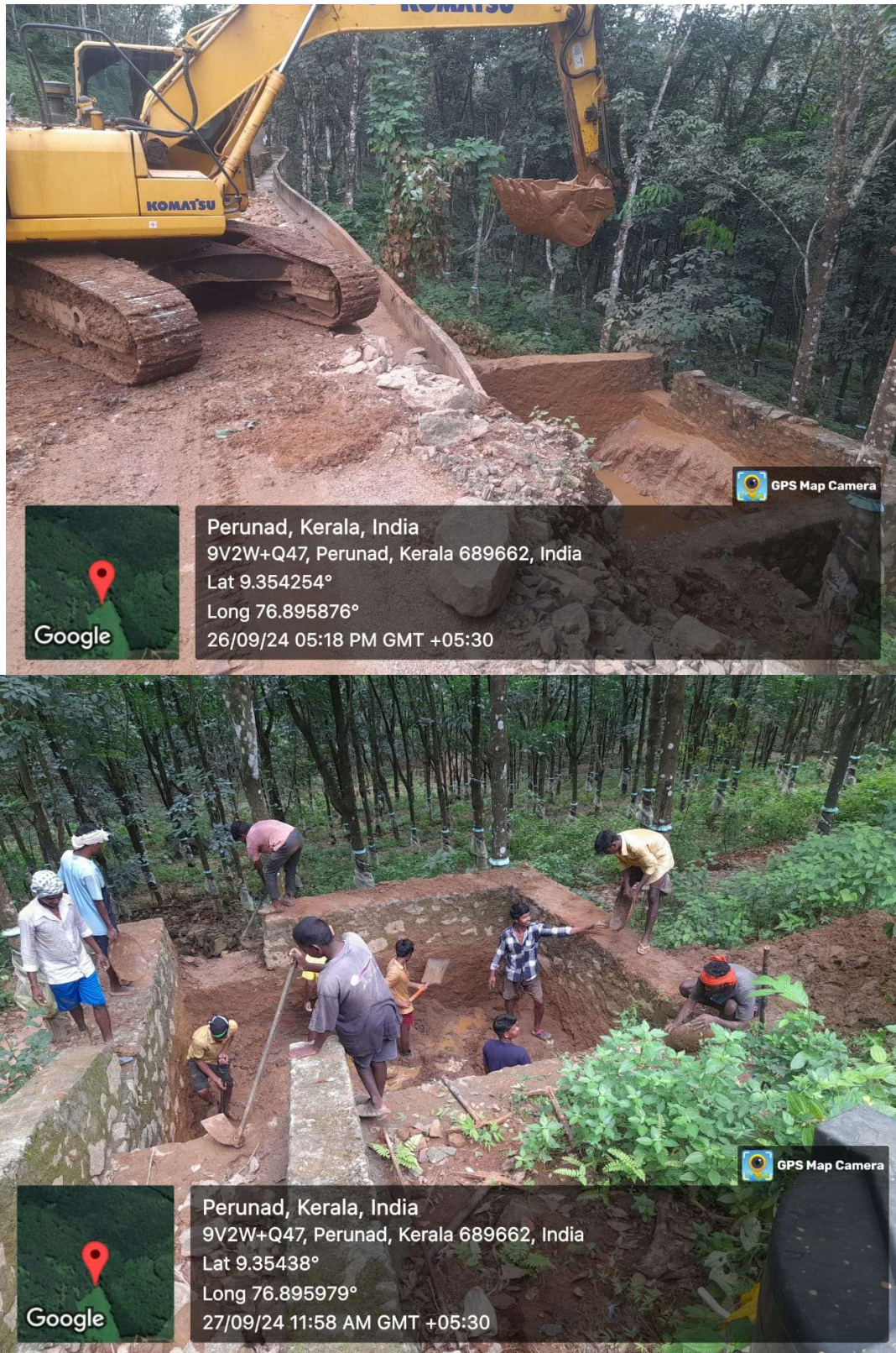
Desilting of traps and Drains
